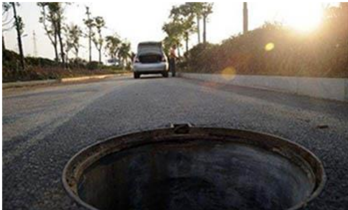
Manholes and manhole covers are everywhere.
